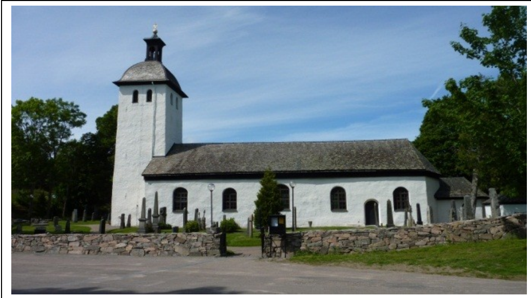
Steneby church, Karlstad diocese in Sweden. Steneby parish has built a bio-fuel central heating for four buildings including the church.
